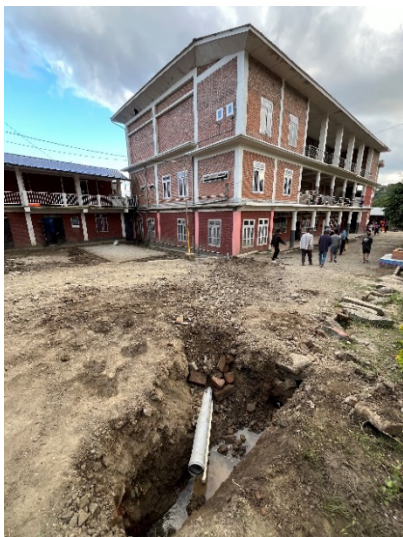
Boys' distribution pipe seen in cream color (lower pipe) & spring water trapping pipe seen in grey color (upper pipe)
