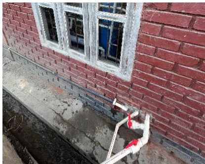
Distribution valve for reject water & boys' drinking area
