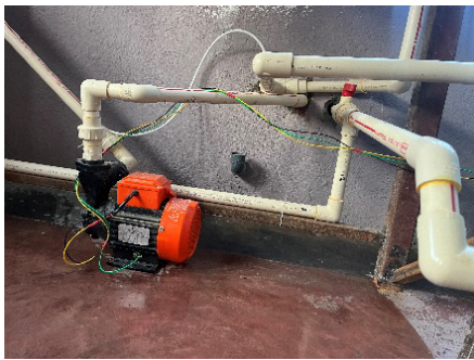
Pressure pump utilize for boys' storage tanks
