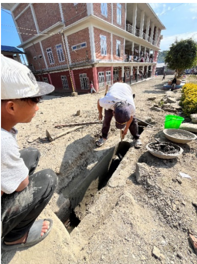
Trapping dam for diverting spring water inside the 26,000 litres cistern
